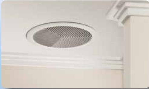
The valve box and ducting are contained in the roof cavity with the ducting connected to a magnetically held, easy-to-clean ceiling grille designed to maximise air flow.
